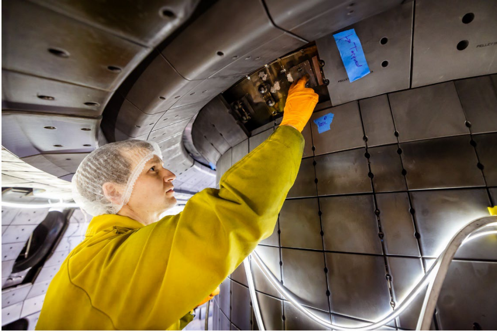
An engineer installs the final protective tiles as part of the Shape and Volume Rise Divertor upgrade
